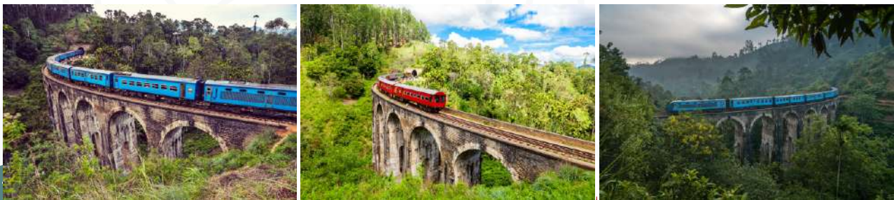
Nine Arches Bridge – Ella
